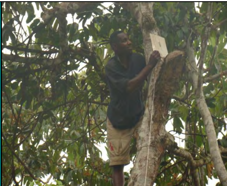
Installation of an artisanal antenna on a tree in Matoto
